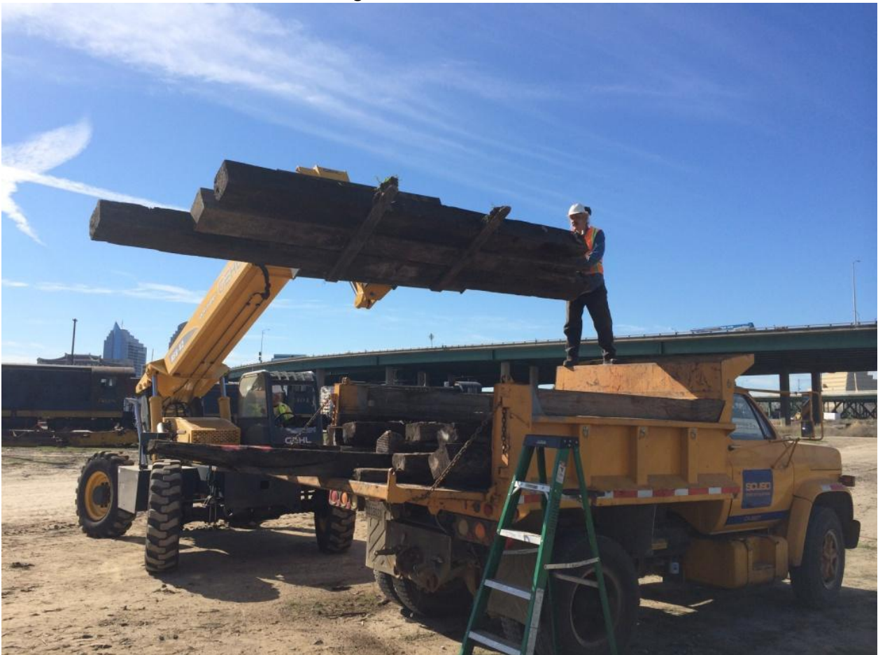
Fred on the dump truck guides Mike F. in the new toy for loading dead ties and timbers
