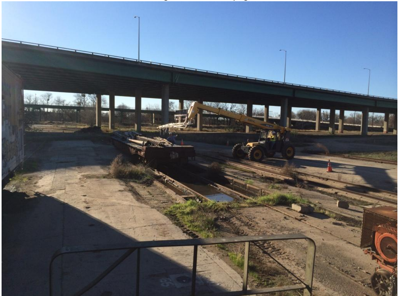
Mike F. extends the grade-all's boom for loading the flat car
