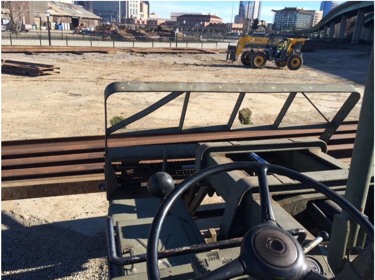
The view from the cab of Big Green while carrying five sticks of 132 lb. rail
