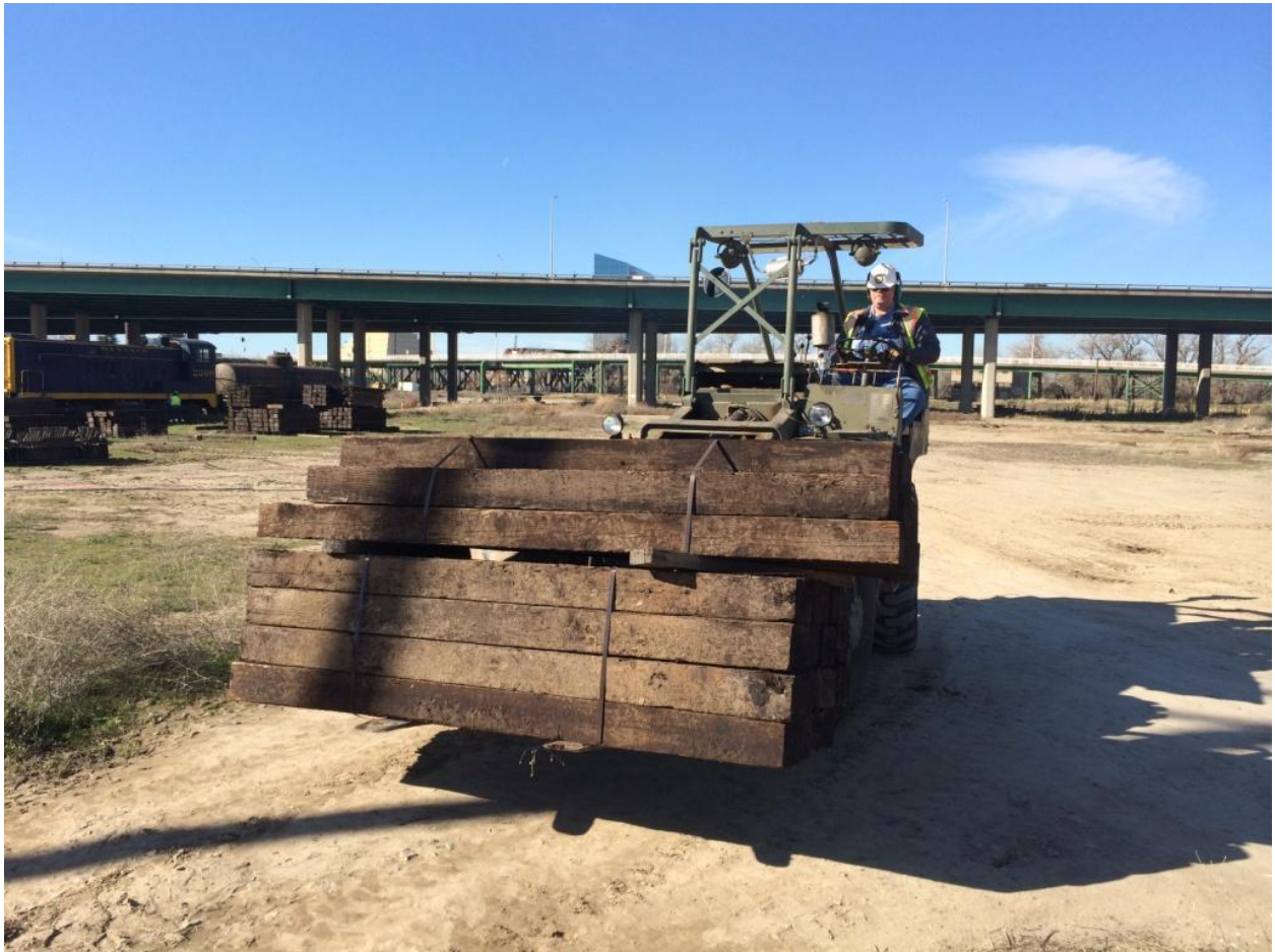
Chris moving two bundles of ties in one load
