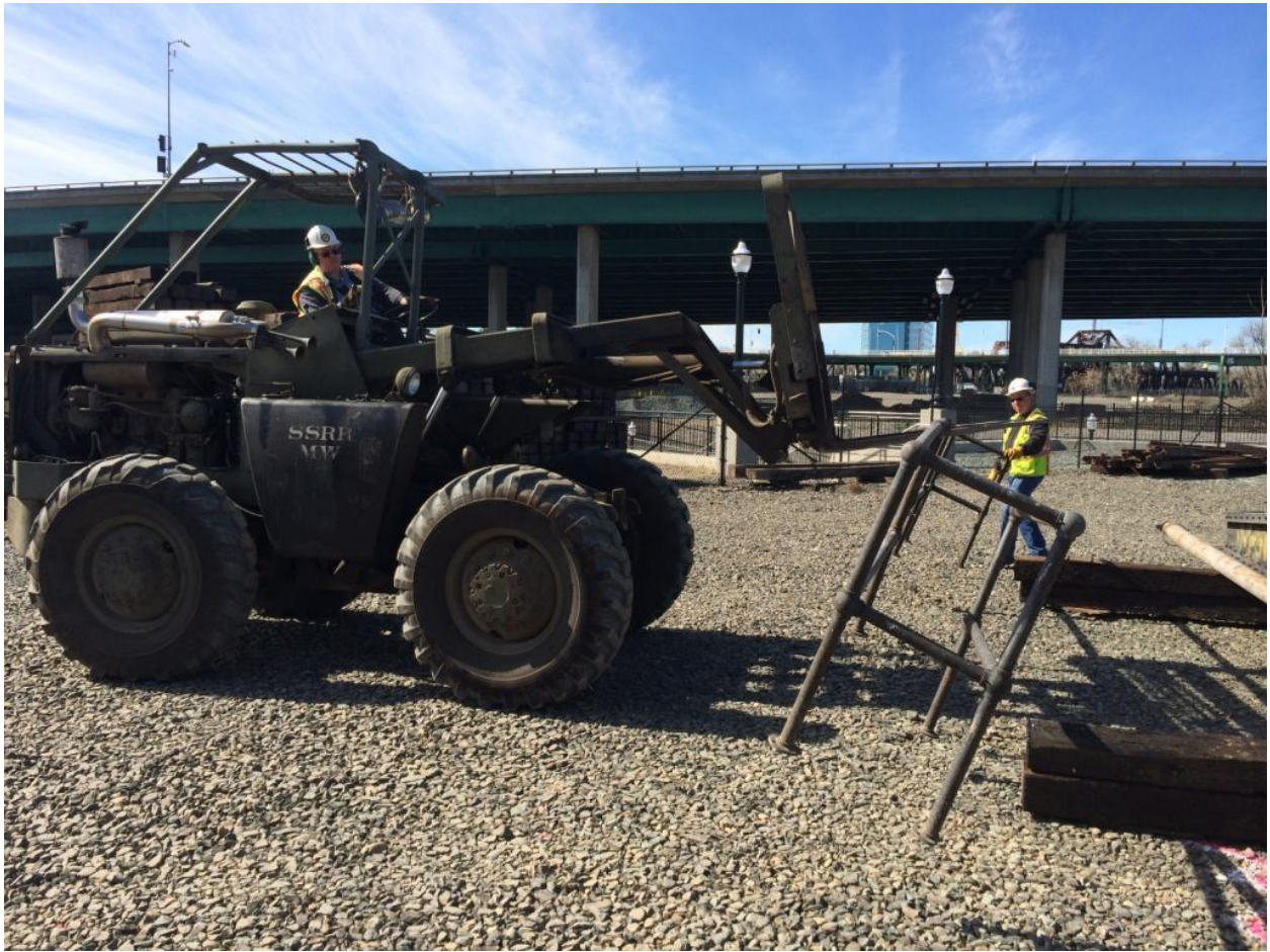
Ed guides in a balustrade that Chris hauled over from the north end of the building
